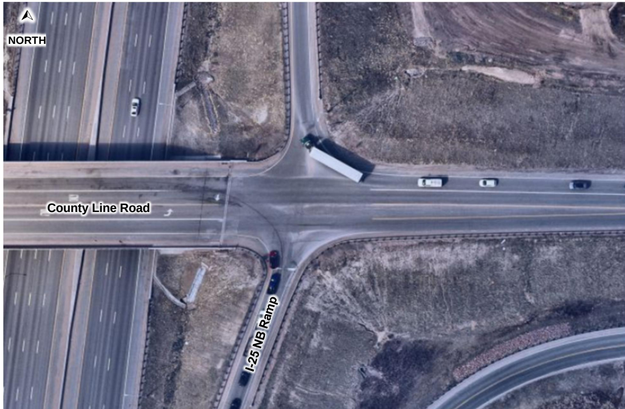
County Line Road & I-25 Northbound Ramp
