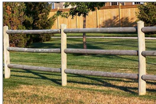
*Figure 38 - Example of Post and Dowel Fencing*
