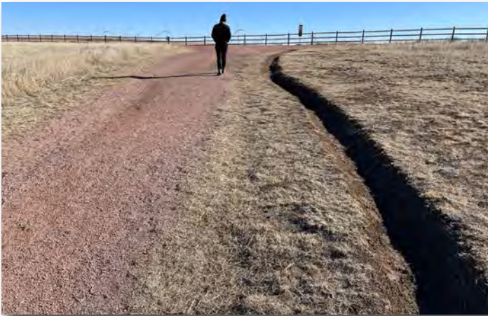
Example of a swale located along an existing trail to direct stormwater away from the trail surface
