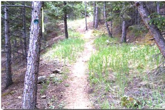
**Tier 4**, 4-foot wide average compacted crush limestone or native soil surface
