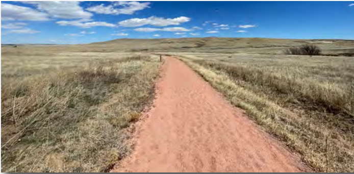
Existing 8' wide crusher fines, looped trail, view looking north
