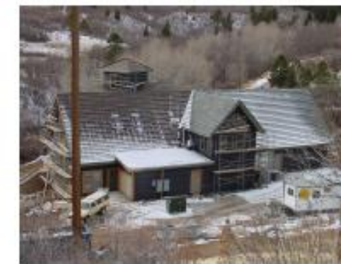
January 5, 2002- Construction continued and the new nature center began to take shape.
