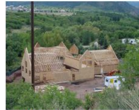
September 8, 2001- During the beginning stages of construction, framing is nearly completed.
