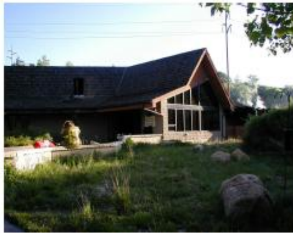
Firefighters worked hard to put out the blaze, however staff offices, educational exhibits, the library, and files and records were all destroyed.
