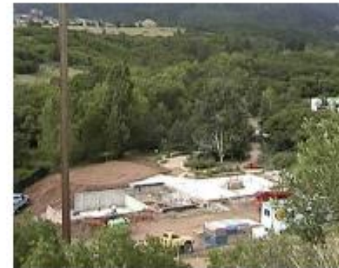
On June 20, 2001, construction began with the use of the original building's foundation footprint. In addition, 4000 square feet of new floor space were added.
