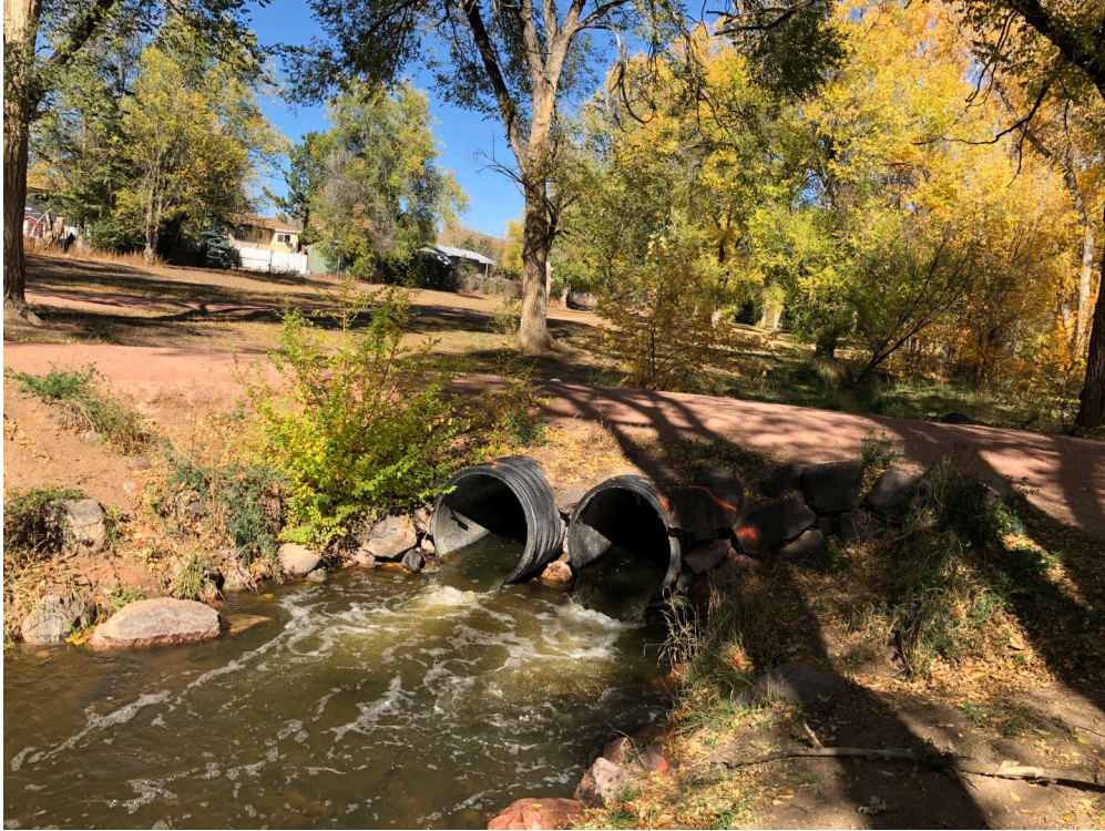
Double culverts where trail crosses Crews Gulch
