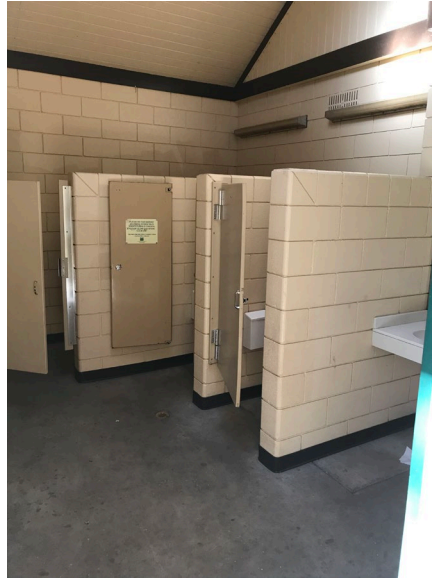
Pine Meadows Women's restroom: 2 sinks, 3 toilets
