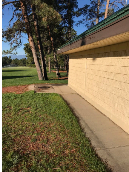
Back of restroom and vault access
