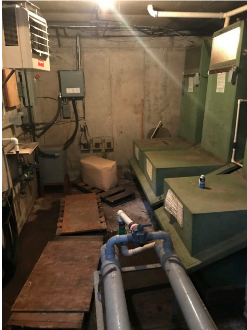
Pine Meadows restroom vault
