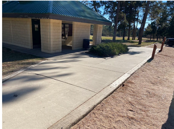
Sidewalk to be replaced and new ADA parking added
