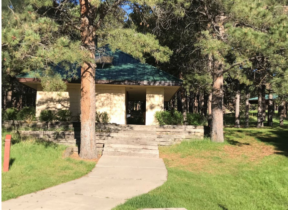
Pine Meadows restroom
