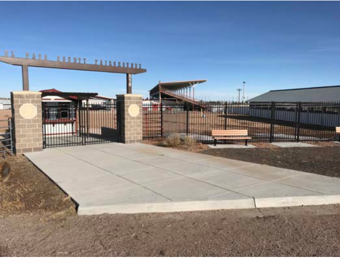
Ticketing booth, start of accessible route
