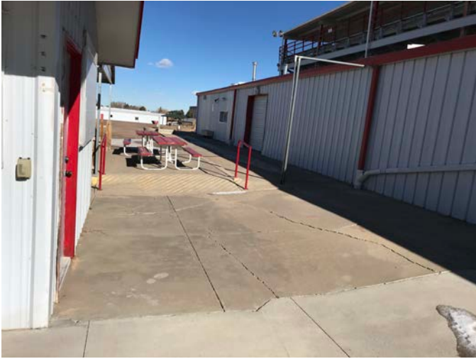
Remove & replace paving, 1
