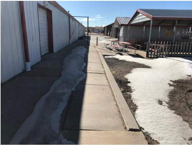
Remove & replace paving, 3. Looking south
