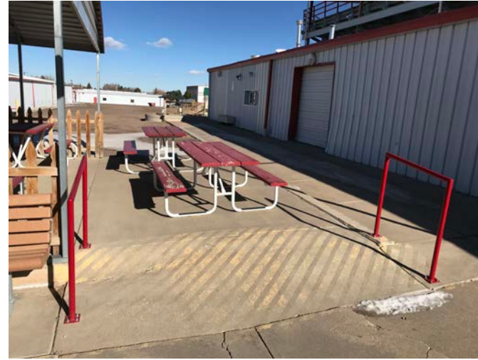
Remove & replace paving, 2
