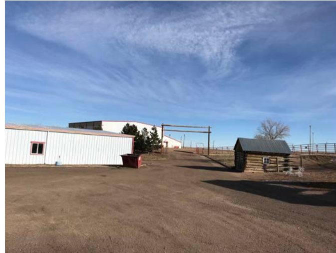
Swink Hall, existing sidewalk to Whitemore building beyond
