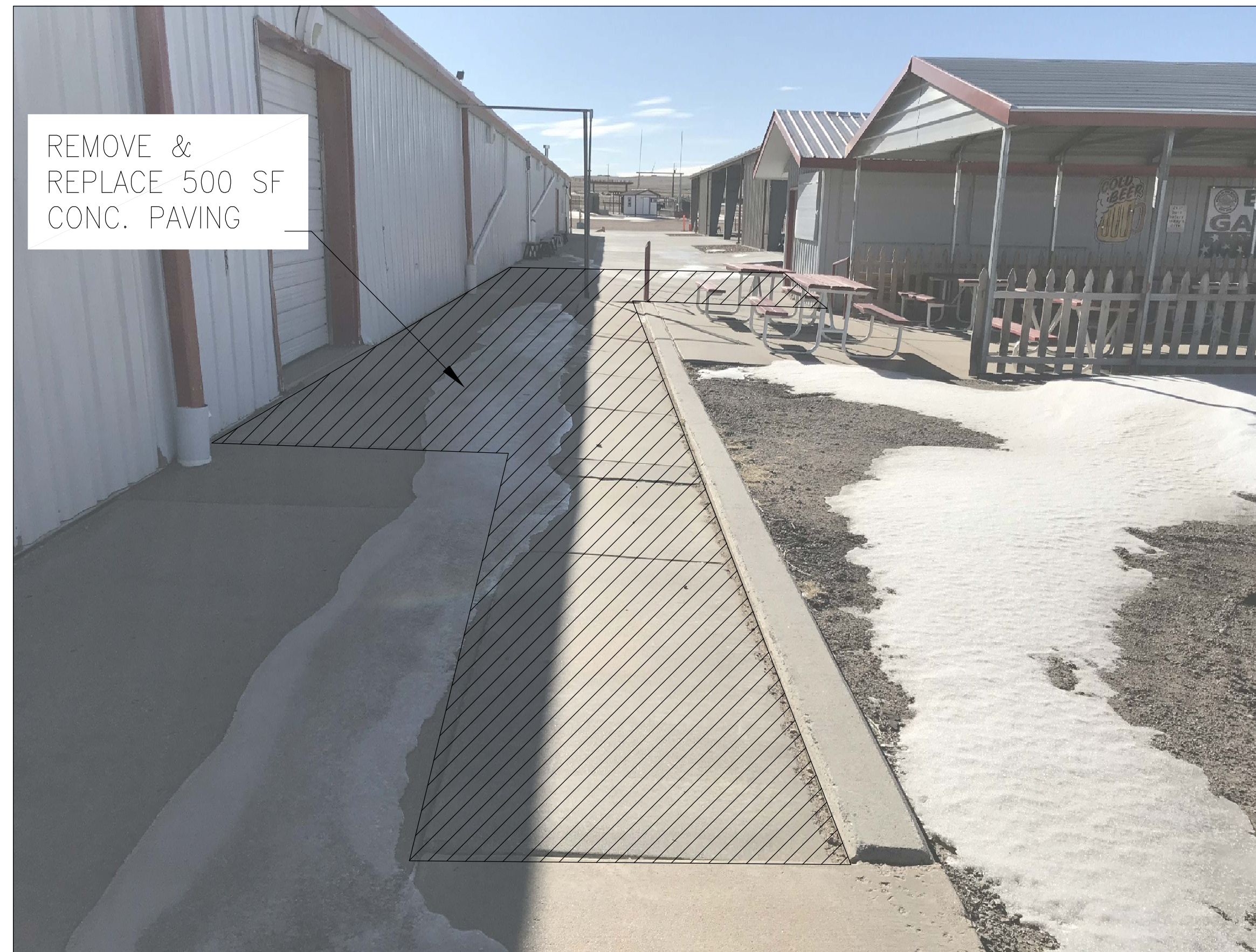
2 REPLACE CONCRETE VIEW 2
