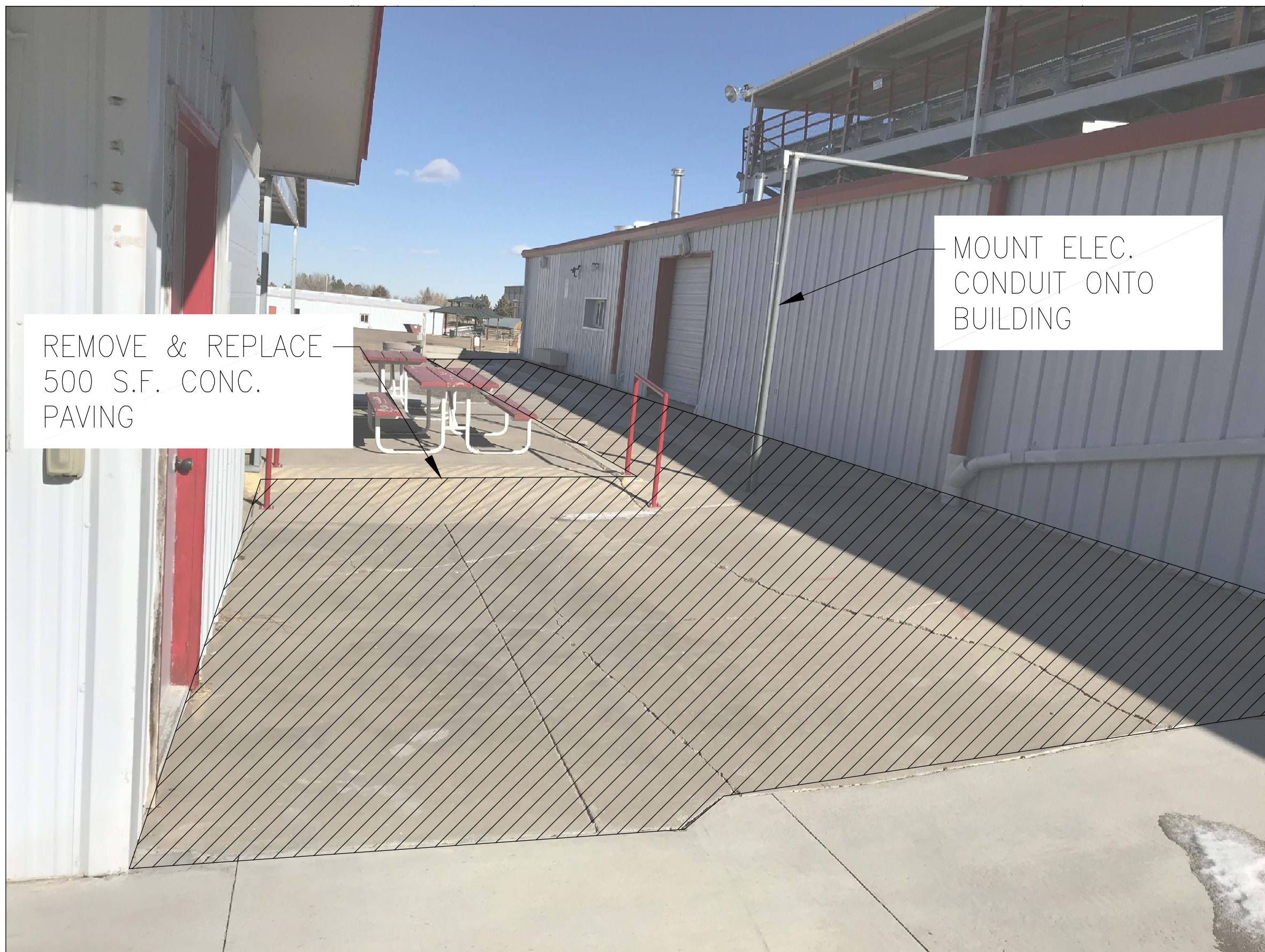
1 REPLACE CONCRETE VIEW 1
