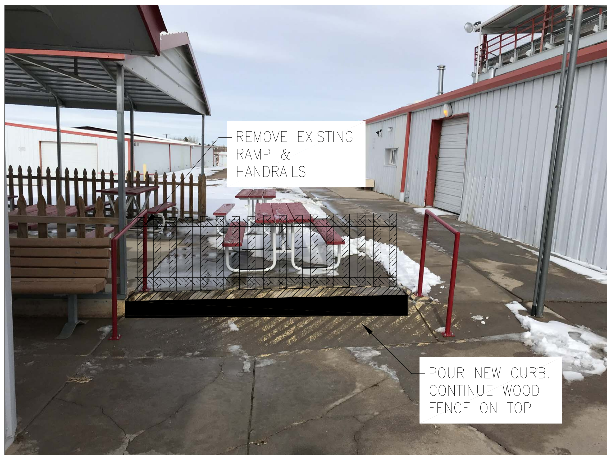
3 REMOVE RAMP & HANDRAILS
