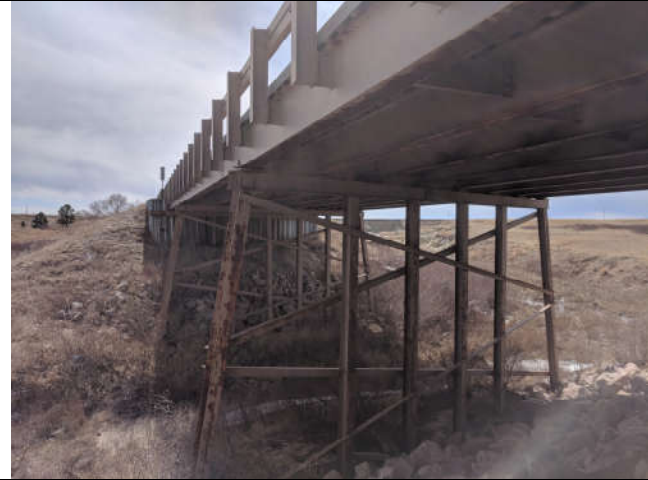
Description: Bridge Underside Direction: South
