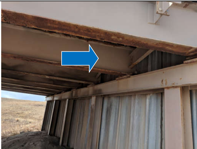
Description: Bridge Abutment (P-Brown, <19ppm Lead) Direction: NA
