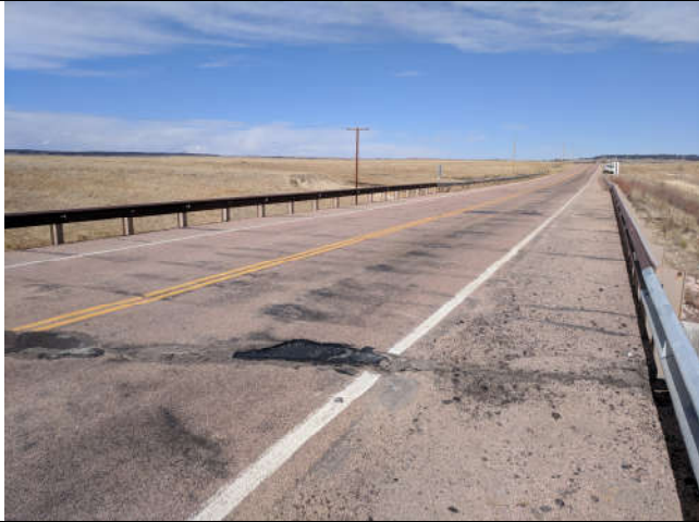
Description: Bridge Deck Direction: North
