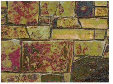
MATCH SHAPE AND AESTHETIC OF COLUMN PICTURED. 6 INCH CONCRETE AROUND BASE OF COLUMN. ROCK IS TO BE COLORADO BLEND LEDGE STONE MATCHING THE COLOR AND AESTHETIC OF NEARBY AMPHITHEATER BOULDERS.
