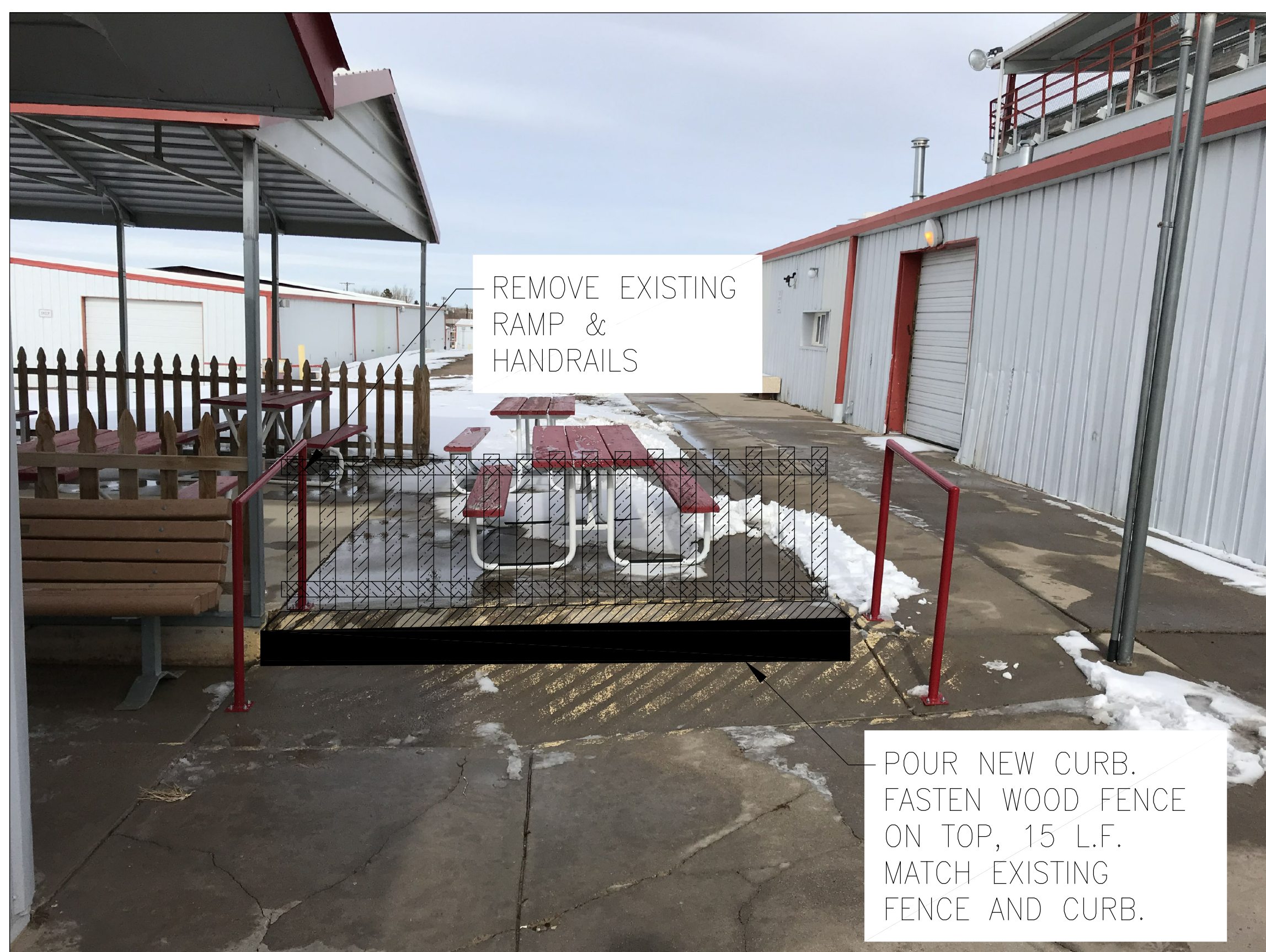
3 REMOVE RAMP & HANDRAILS
