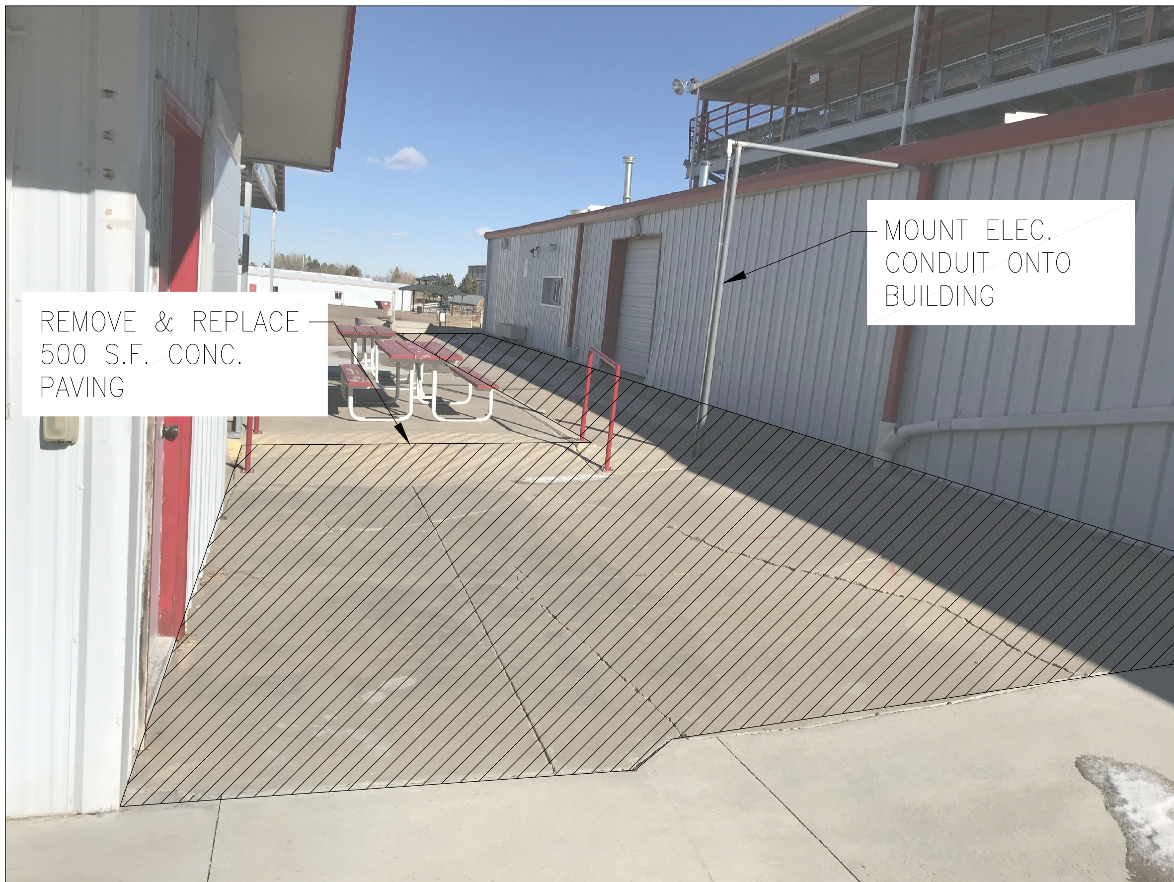
1 REPLACE CONCRETE VIEW 1
