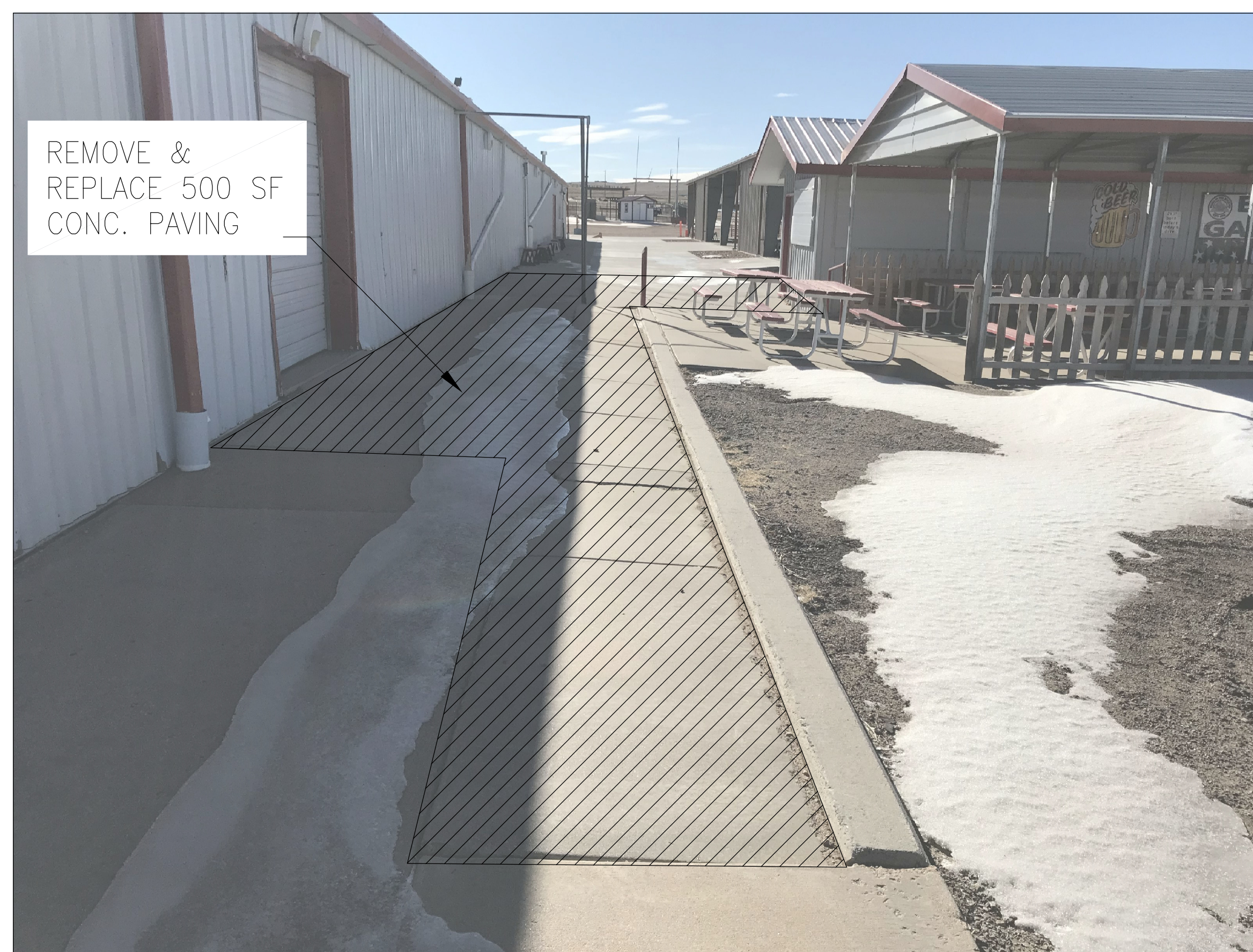
2 REPLACE CONCRETE VIEW 2
