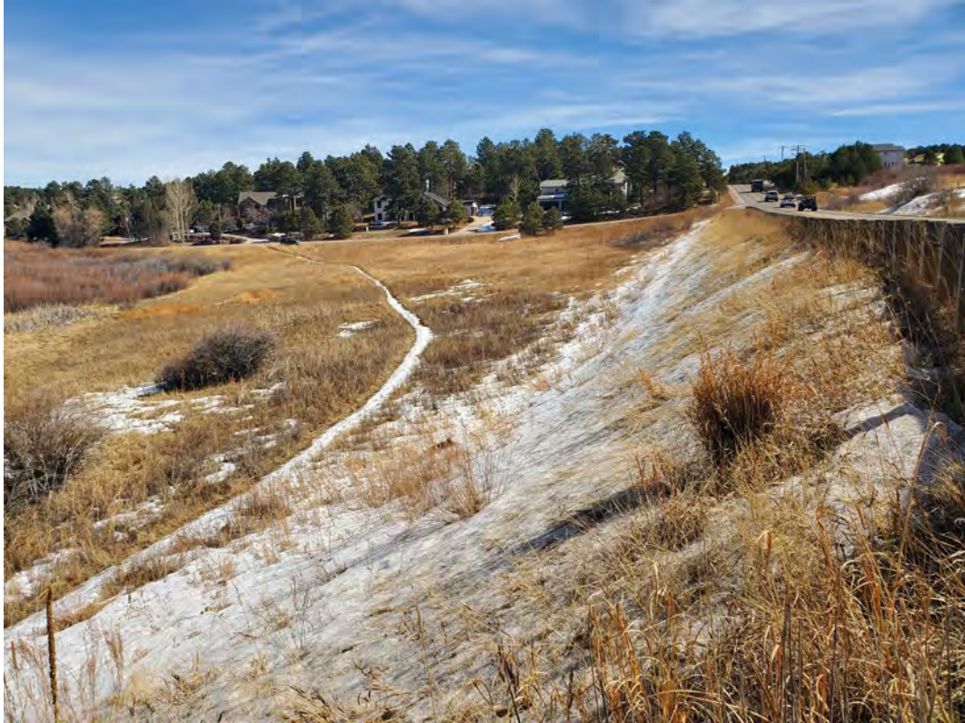
Photo 7. View looking east along the north side of Highway 105 at the location of the proposed retaining wall. The habitat to the north of the wall be protected.
