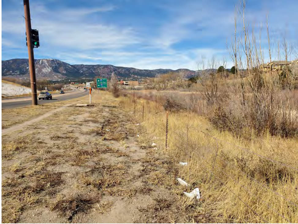
Photo 1. View looking west along the ROW adjacent to the CDOT conservation property, which is located to the right of the barbed wire fence. The disturbance along the roadside is evident.
