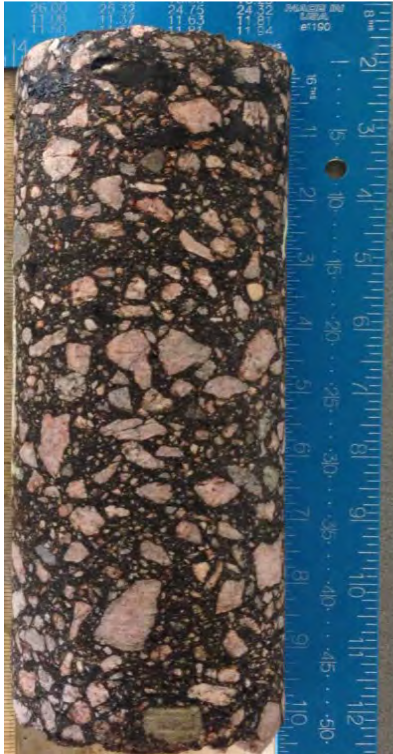
Pavement Core at SW-P-02 Westbound lane. 10 inches thickness measured
