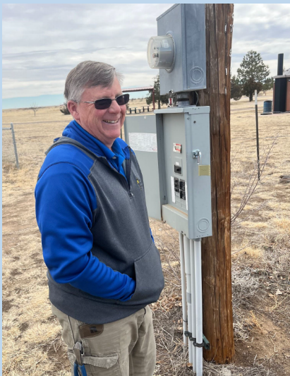
Glenn Wilson, of Glenn Wilson Electric, upgraded electrical panels at Kirk Hanna Park.
